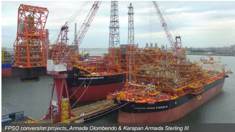
FPSO conversion projects, Armada Olombendo & Karapan Armada Sterling III
