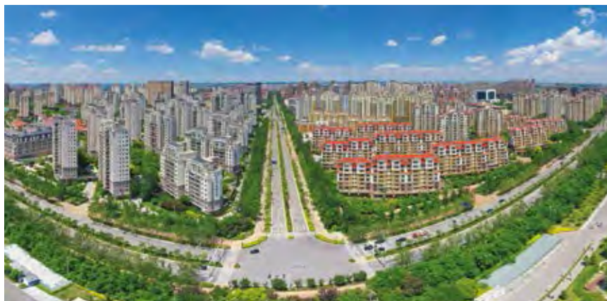
Development of the Eco-City continued in 2020 with the sale of two residential land plots in the Central and South districts.
