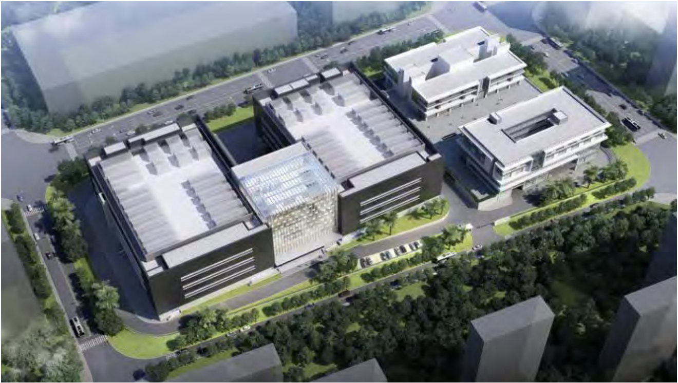
Alpha DC Fund entered into the fast-growing data centre market in China with the development of a greenfield data centre in Tonghu Smart City in Huizhou, Guangdong.
