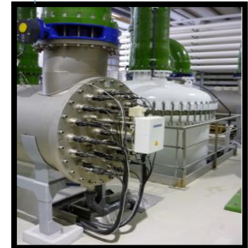
UV as primary disinfection process
